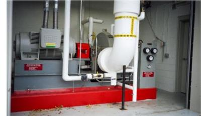
A small condensing unit is fuelled by scrap wood helping a crate manufacturer reduce its total energy costs. 1 MW Synchronous Unit.
